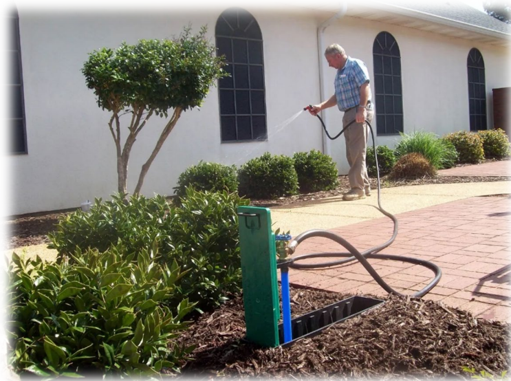
Hose connections for maintenance staff at pedestrian bench locations.
