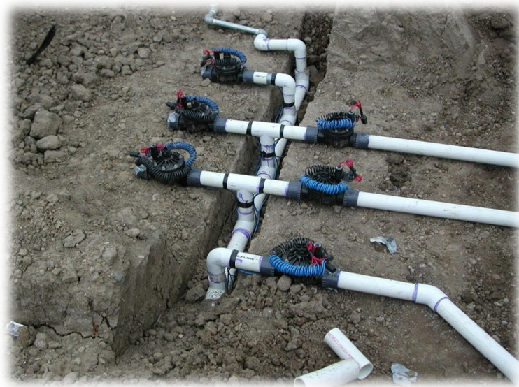
All new irrigation components need to be installed.
