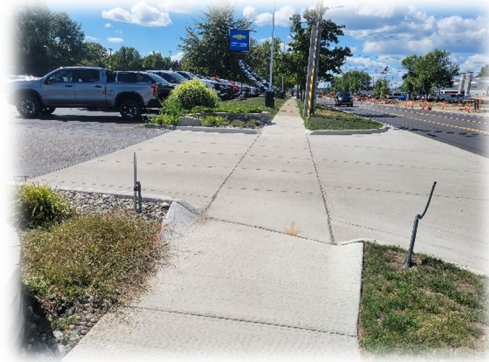
Existing system pipe has been abandoned.
