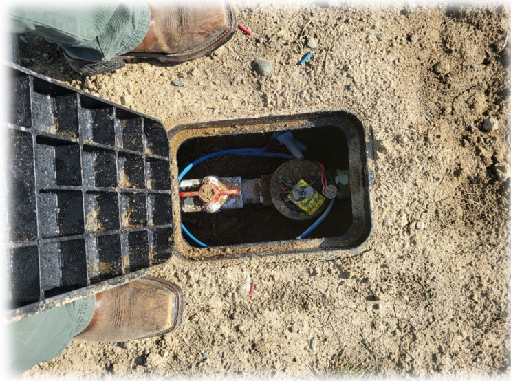
Zone valve installation with rectangular valve box, manual valve, waterproof wire splices, two-wire cable, and zone identification tag.
